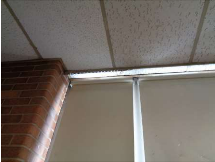
Photograph 5: Rusted ceiling tile tracks in Classroom A-5.
