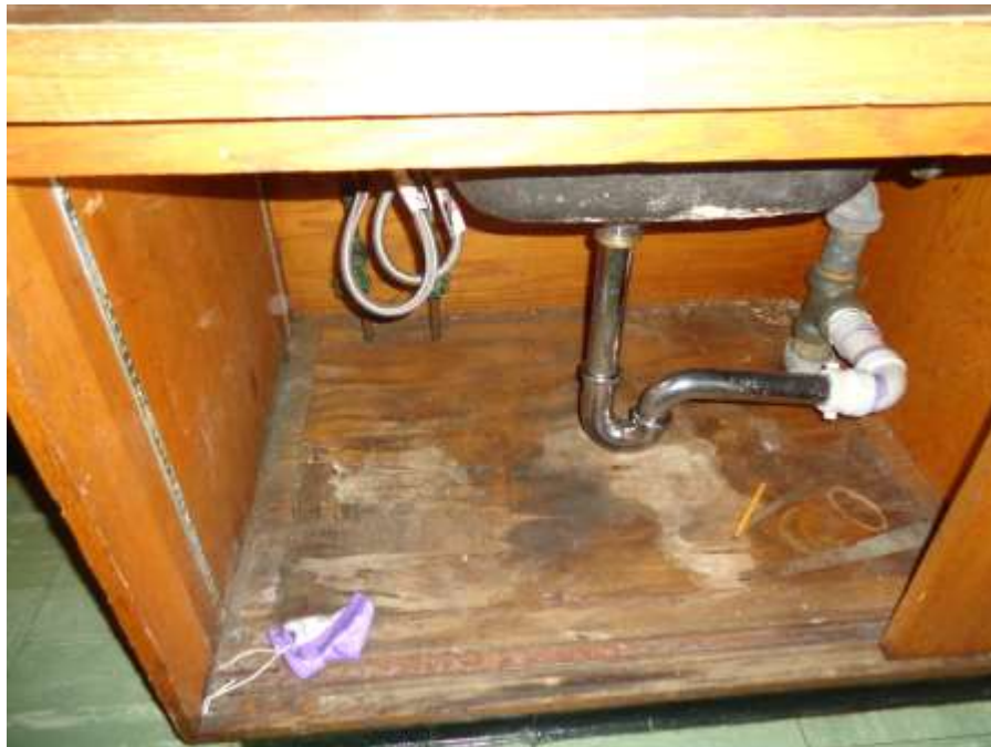
Photograph 3: Wood shelving below classroom sink in Room 26.
