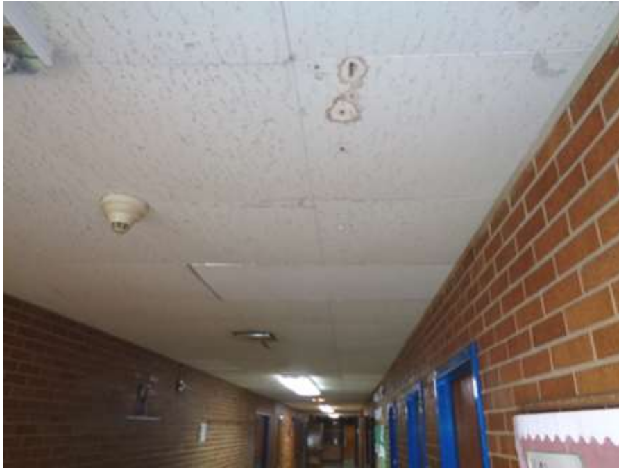
Photograph 1: Ceiling Tiles in 1st Floor Hallway.
