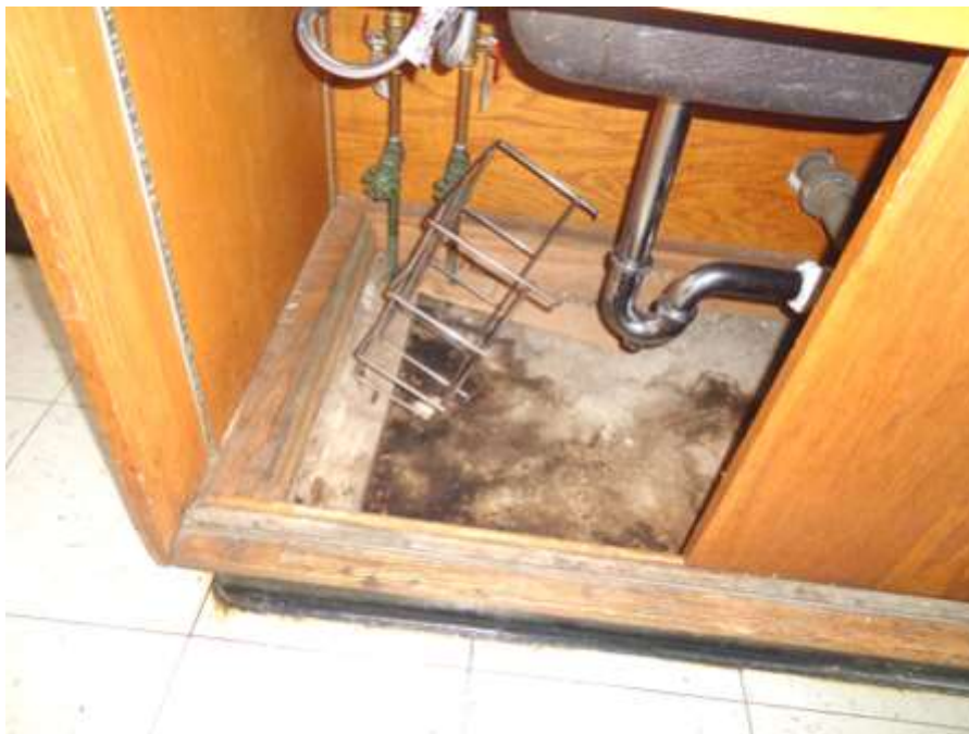
Photograph 2: Wood shelving below classroom sink in Room 28.
