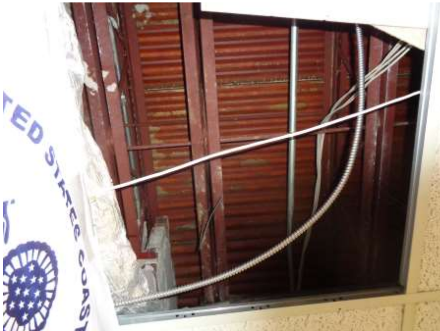
Photograph 6: Evidence of water intrusion above ceiling tiles.
