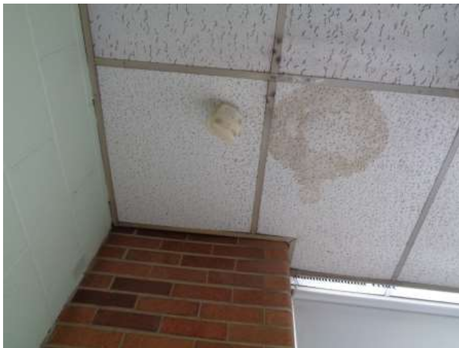
Photograph 4: Example of water damage on ceiling tiles in classrooms.
